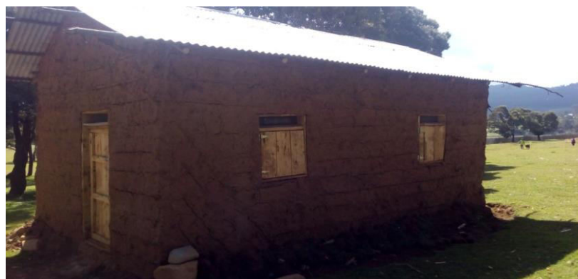
Figure.1 Warehouse, for storage of potato tubers
